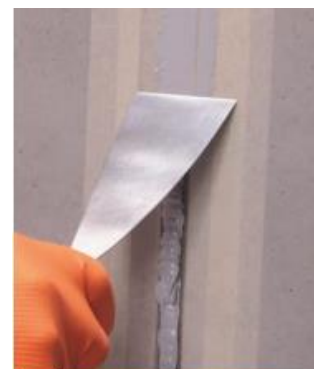
Smoothing over Mapeflex PU40
